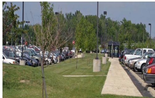
Park and Ride facility in the City of Mentor.
