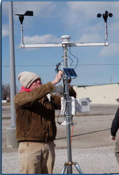
Weather station installation at Perkins
