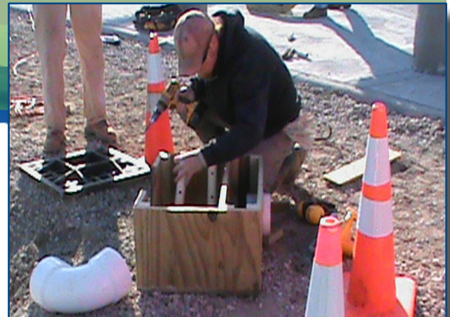
Monitoring installation at Perkins Township facility
