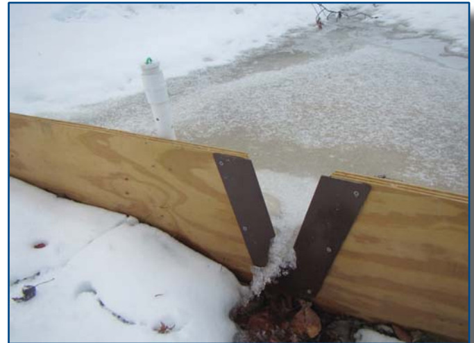
Ice behind weir, Orange Village
