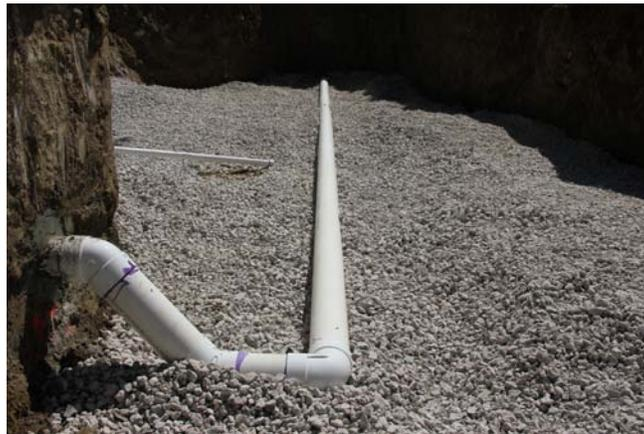
**Figure 5:** The underdrain with an upturned elbow provides an internal water storage (IWS) zone within the bioretention cell at Holden Arboretum.
