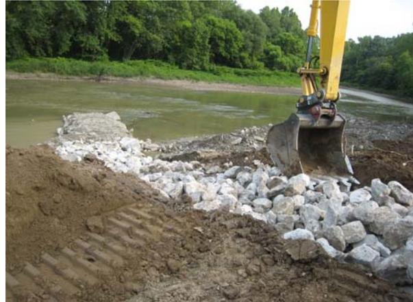
To prevent the river from cutting behind the weir, each weir has a key (stone filled trench) that continues up the slope.
