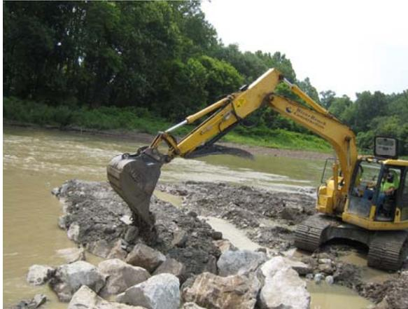
Bendway weirs are constructed by placing the largest rocks first, and then placing smaller and smaller rocks in the gaps until each weir is complete.
