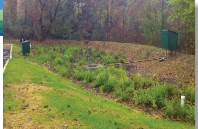
*Bioretention cell installed at the edge of parking lot with installed monitoring equipment at Ursuline College.*
