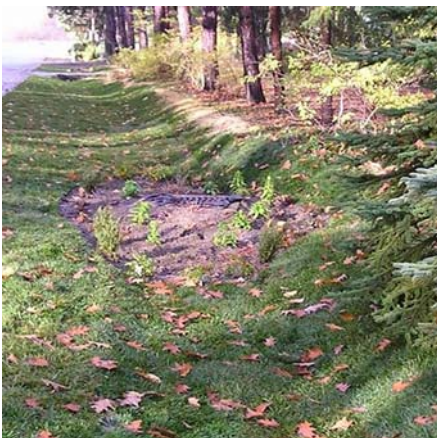
After: Bioretention swales with rain garden inserts manage stormwater at its source.
