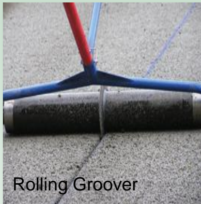
Improper Porous Concrete Installation
