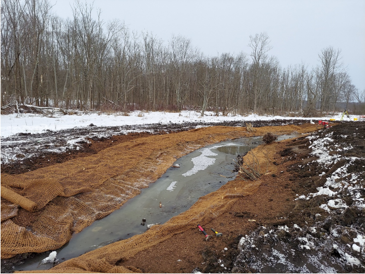
Figure 4. Beaver Creek Restoration Project during construction. Photo source: BioHabitats, February 2021.
