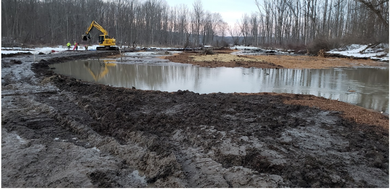
Figure 6. Beaver Creek Restoration Project during construction. Photo source: BioHabitats, February 2021.
