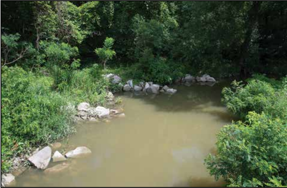
Above: New bendway weirs protect the stream bank upstream of hole 18. Below: Construction at hole 13 involved rerouting a section of the stream away from a heavily eroded embankment, which was reinforced with rock.
