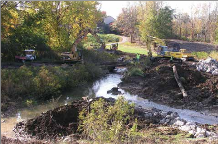
Above: New bendway weirs protect the stream bank upstream of hole 18. Below: Construction at hole 13 involved rerouting a section of the stream away from a heavily eroded embankment, which was reinforced with rock.
