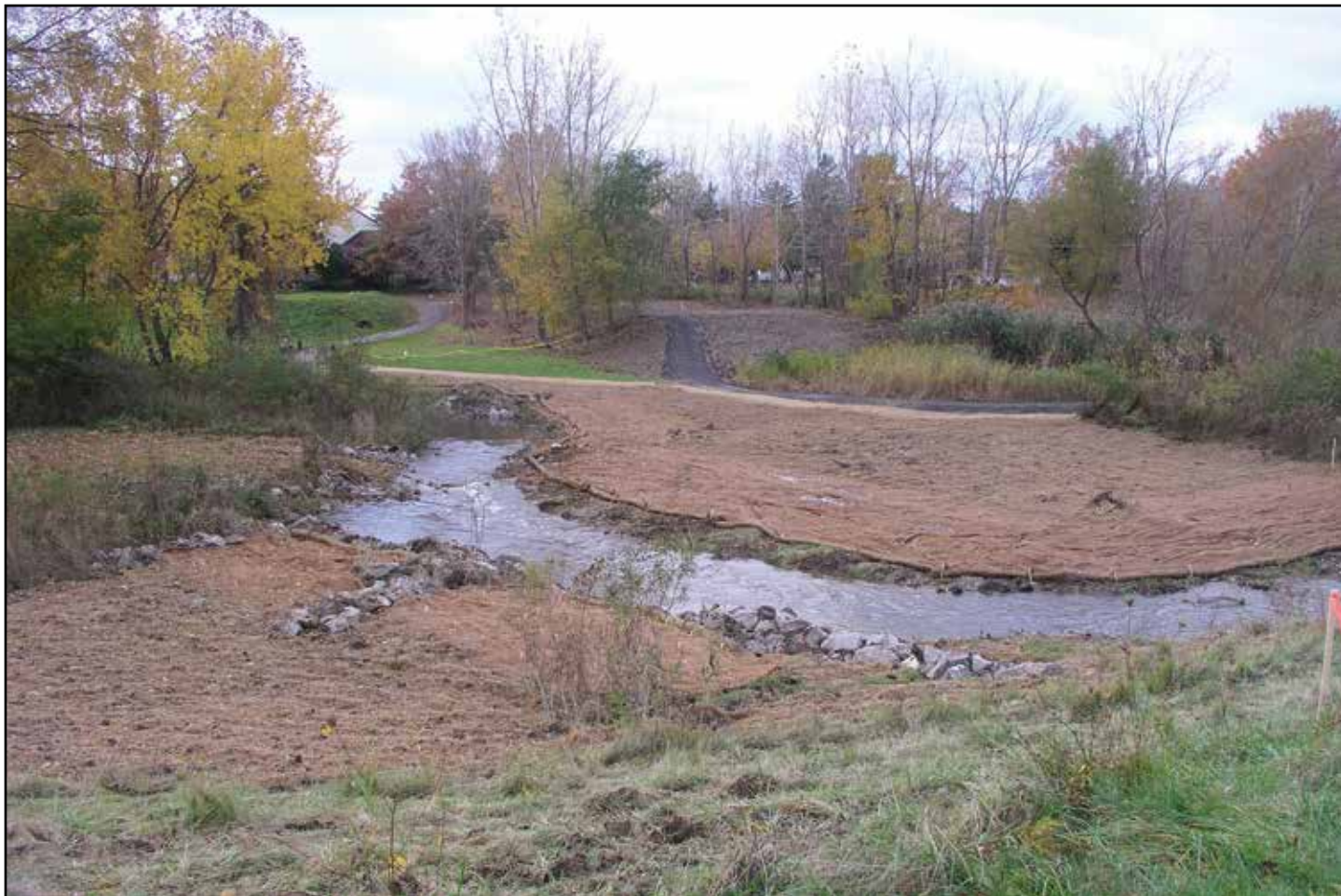
Erosion control matting at hole 13 kept soil and fledgling plants in place through the winter in the newly excavated riparian flood plain.
