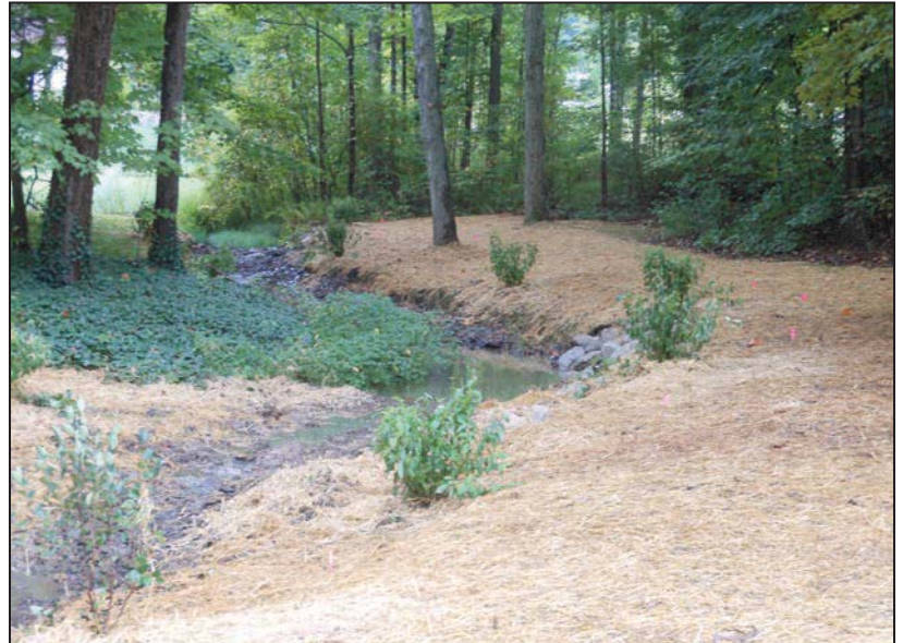
Stabilized streambanks on residential property in Kirtland
