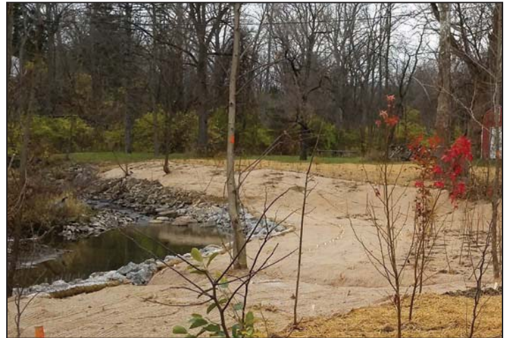
Solon stabilized Hawthorne Creek's stream channel and restored floodplain access
