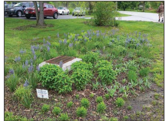
Bioretention cell
