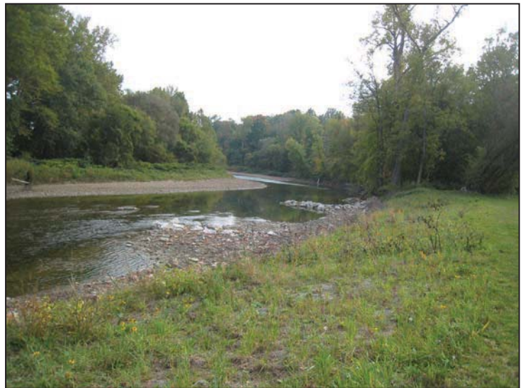
Bendway weirs on Chagrin River's Main Branch at Todd Field in Willoughby
