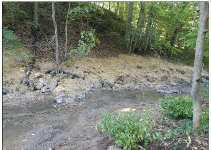
Stabilized streambank on residential property in Munson Township
