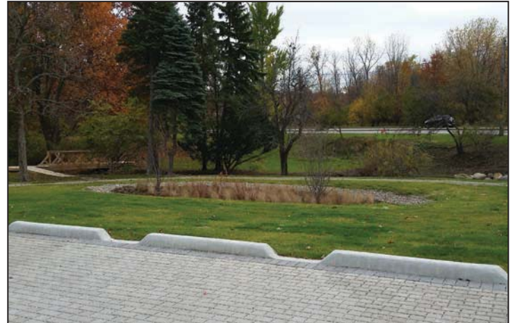
Permeable pavers drain to a rain garden at Morgan Park in Pepper Pike to treat runoff to a Pepper Creek tributary
