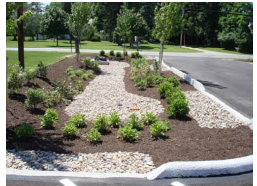
Bioretention cell after planting
