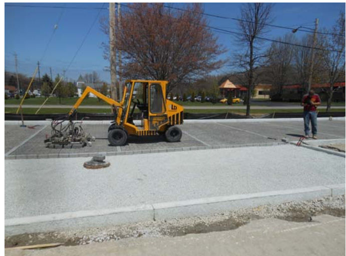
Pavers being installed over gravel and stone layers
