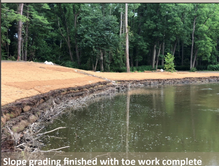
Rootwads installed, begin back fill of toe
