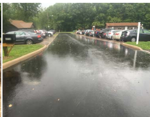
Permeable pavement at Centerville Mills Park installed in 2016.
