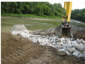
Bendway weirs need to be keyed into the bank to prevent the river from cutting behind them.
