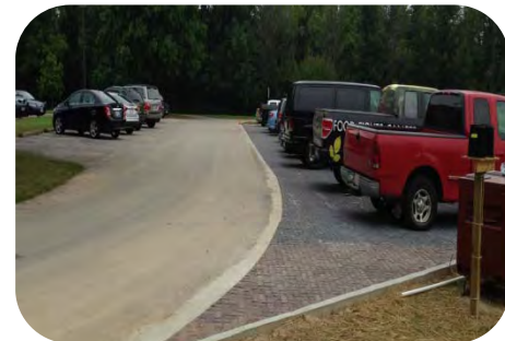
Old Woman Creek NERR Permeable Interlocking Concrete Pavers
