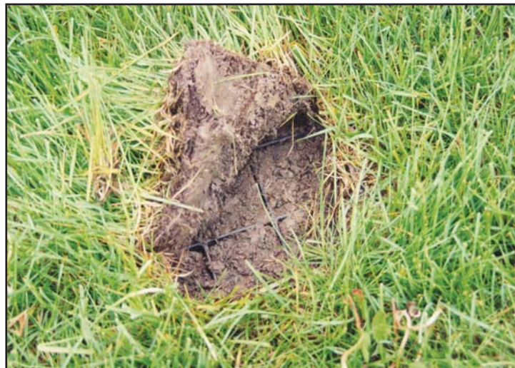
Figure 2.11.9 Vegetated Grid System with established turf grass.
