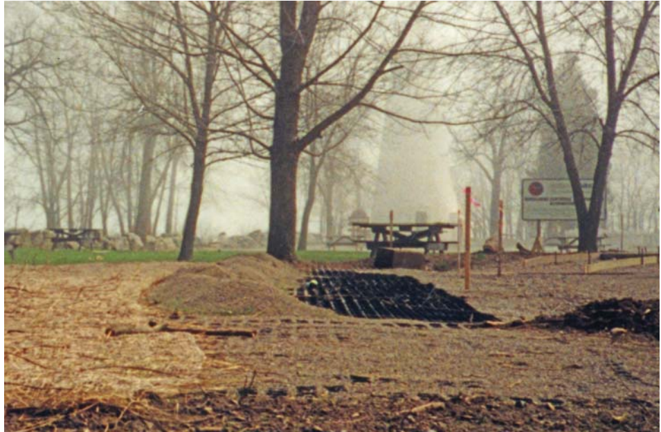
Pervious Paver installation
