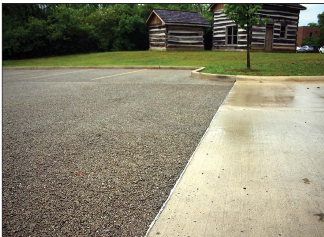
Figure 2.11.1 Porous Concrete at Indian Run Park in Dublin, Ohio.
