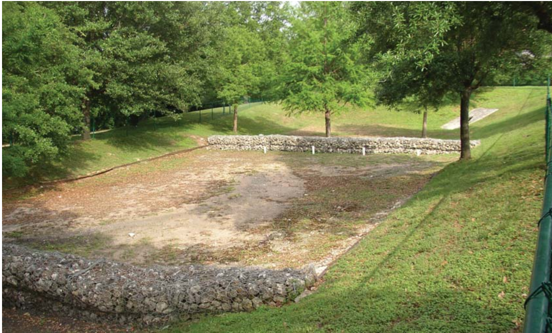
Above-ground Austin Sand Filter and sand filtration chamber.
