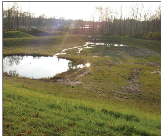
Figure 1. "Dry" extended detention pond with a forebay and a micropool (near the dam and the outlet).
