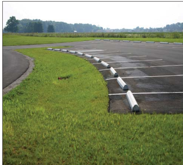
Figure 2. Disconnecting parking and storm sewers in order to reduce pollutant loads.
