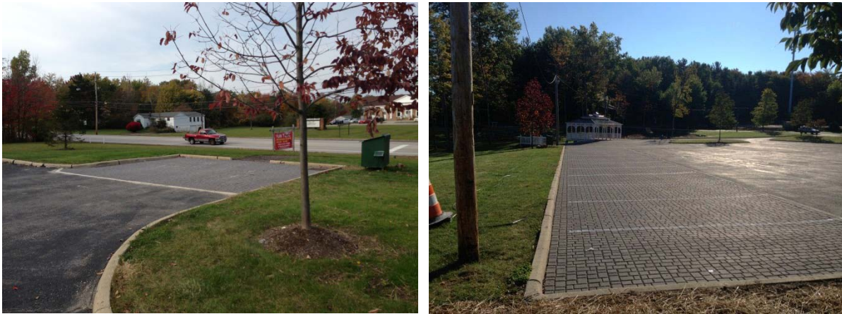
Figure 5. Small (left) and Large (right) permeable pavement applications at Willoughby Hills.
