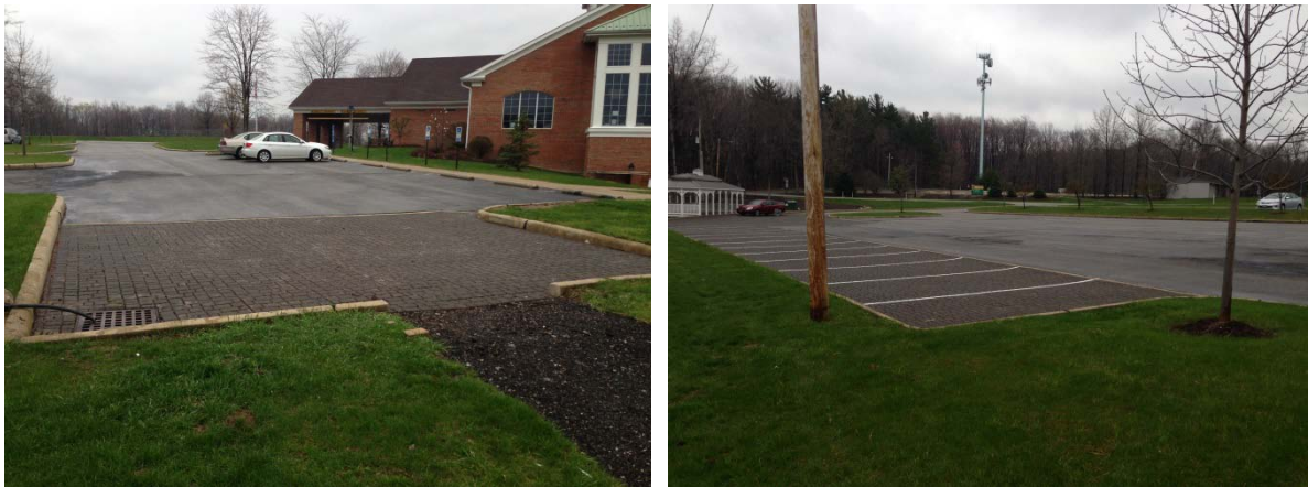
Figure 34. Small (left) and Large (right) permeable pavement applications at Willoughby Hills, Ohio community center.
