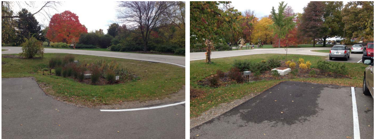
Figure 22. Photographs of the Holden Arboretum South (at left) and North (at right) bioretention cells 13 months post-construction.
