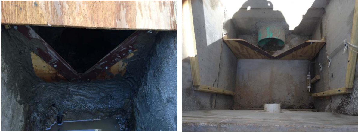
Figure 25. Weir installed in the outlet structure of the south bioretention cell at Holden Arboretum (left) and top view of weir installed in Ursuline College outlet structure (right).
