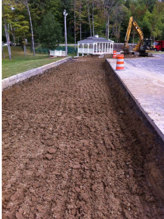
Figure 38. Raked soil at the bottom of the subgrade at Willoughby Hills.
