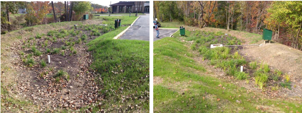
Figure 20. Photographs of the Ursuline College bioretention cell six months post-construction.
