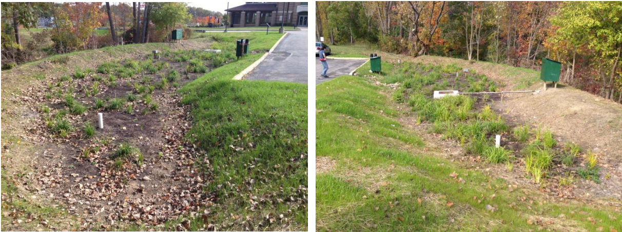
Figure 51. Photographs of the Ursuline College bioretention cell six months post-construction.
