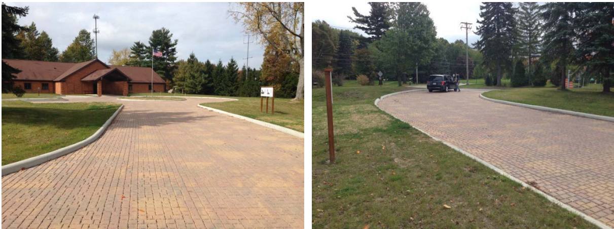
Figure 7. Photos of the Orange Village PICP parking lot.
