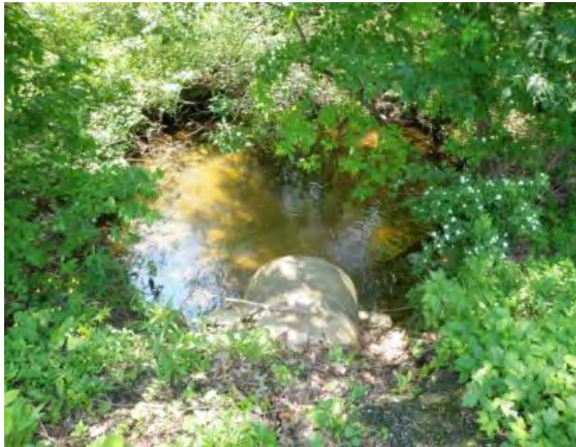
Figure 60: Scour pool at culvert downstream of Wyandot Road
