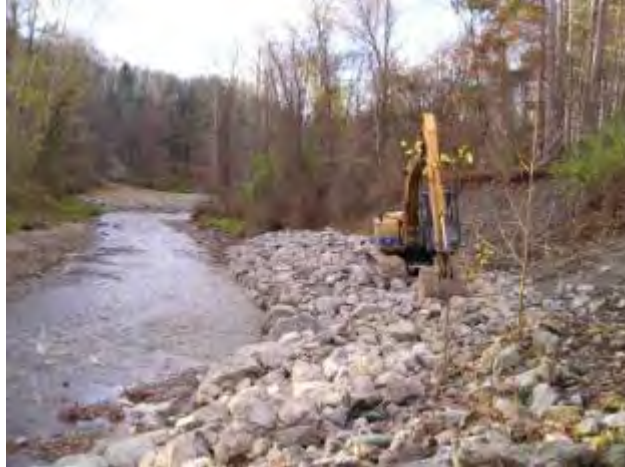
Figure 54: ODOT Repairs Near Crowley Bank Stabilization
