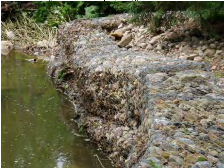
Figure 52: McNitt Property 2010, gabion structures
