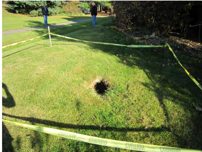
Sinkhole developing at Burlington Green subdivision from failed pipe.
