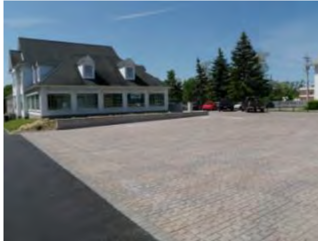
Figure 58: Permeable Pavers at 8555 Mayfield Road, Chester Township
