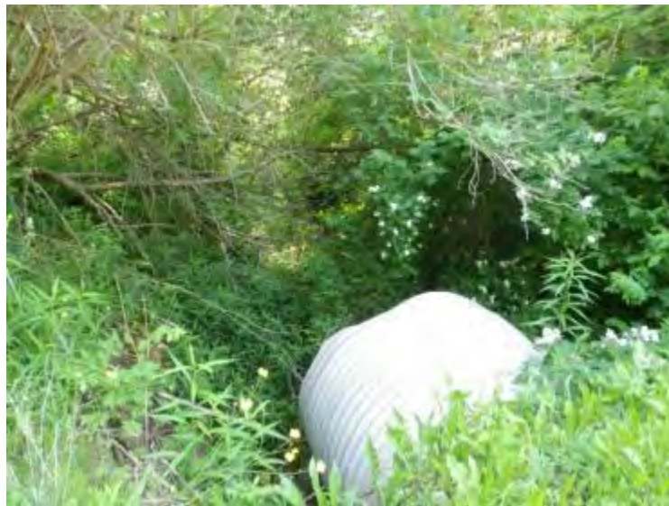
Figure 62: Heavy vegetation downstream of culvert, Ranch Drive
