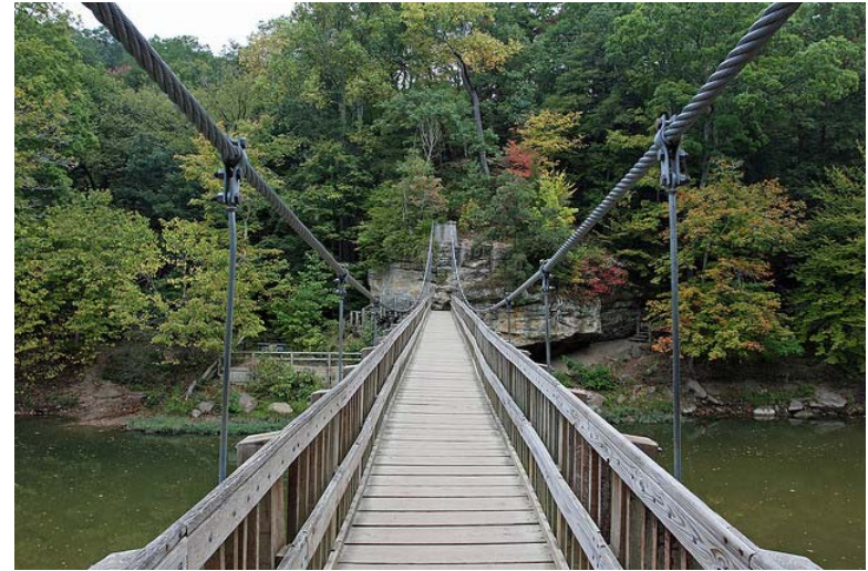
Simple Suspension Structure
