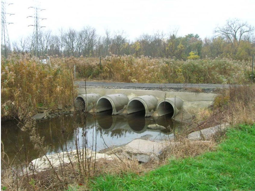
Existing Drainage way Culvert
