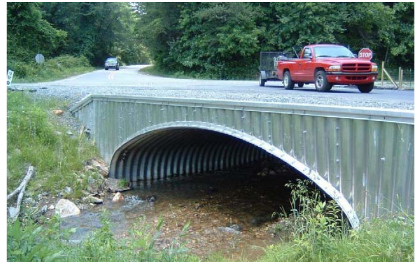
Metal Culvert Structure
