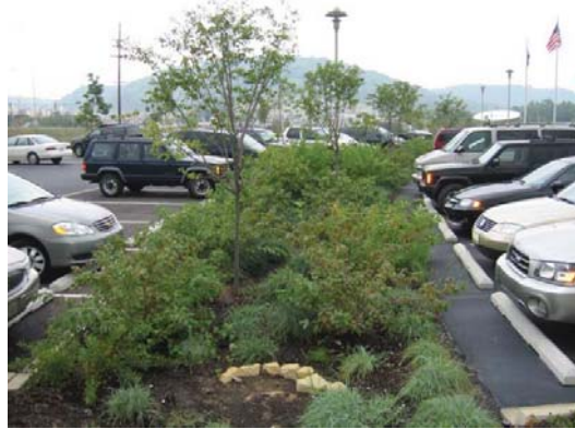
Stormwater Bioswales
