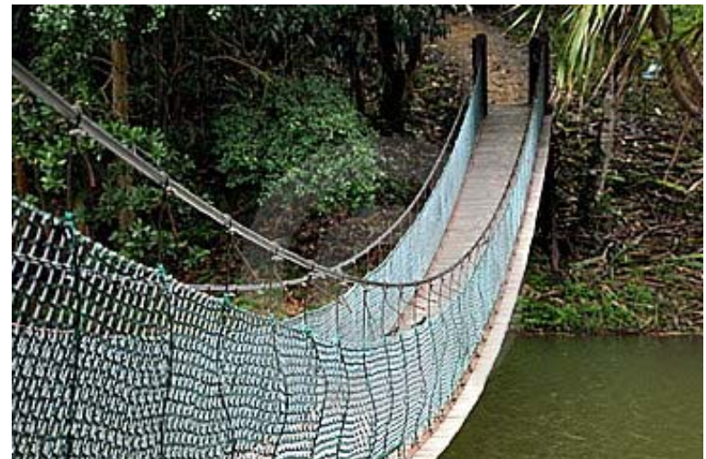
Simple Suspension Structure
