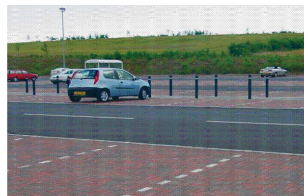
Compact car spaces on pervious pavement
