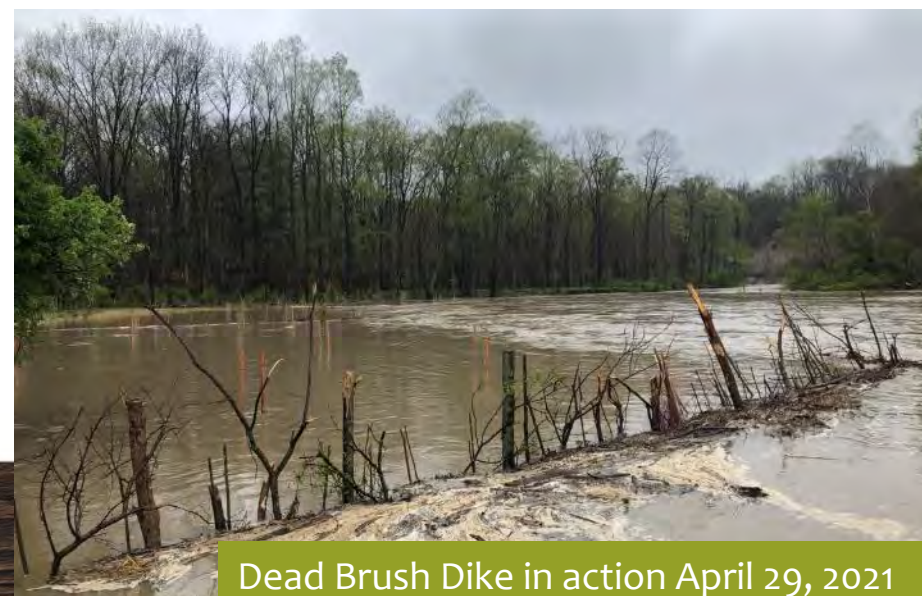
Meander logs w/ dead brush dike in background
