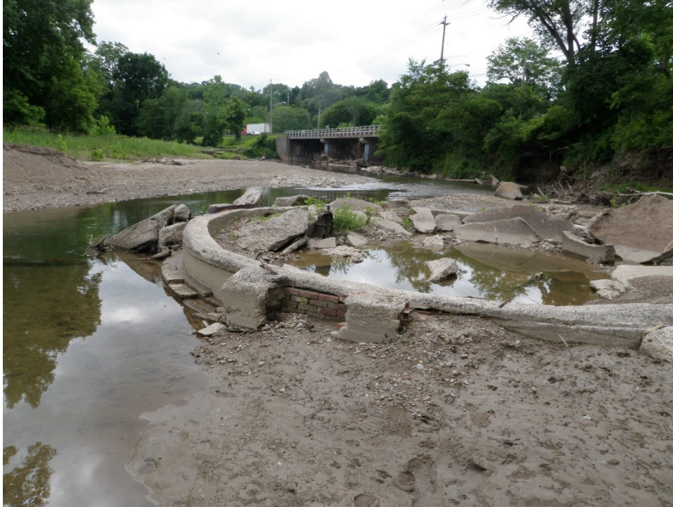
Figure 6. Former City water intake structures contribute to erosion and sedimentation at the mouth of the East Branch. Photo source: Chagrin River Watershed Partners, June 26, 2018.
