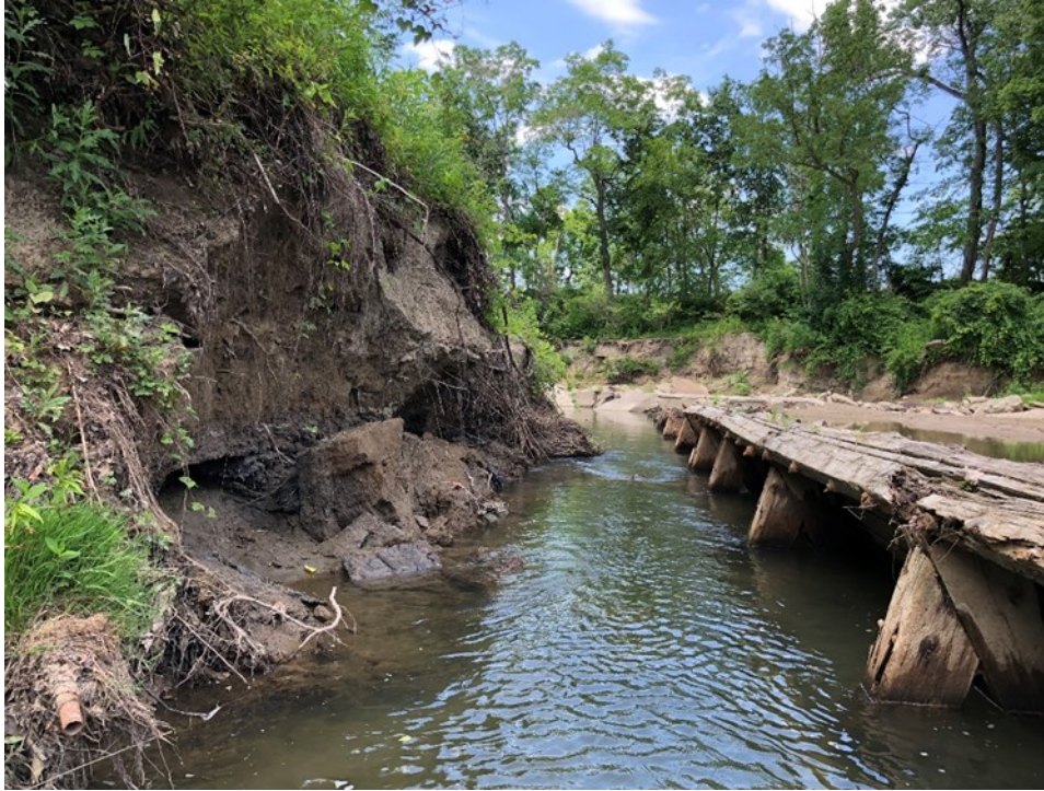
Figure 7. Former City water intake structures contribute to erosion and sedimentation at the mouth of the East Branch. Photo source: Chagrin River Watershed Partners, June 26, 2018.
